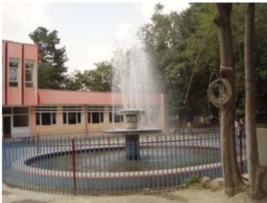
Behind the new fountain is the future education building.
